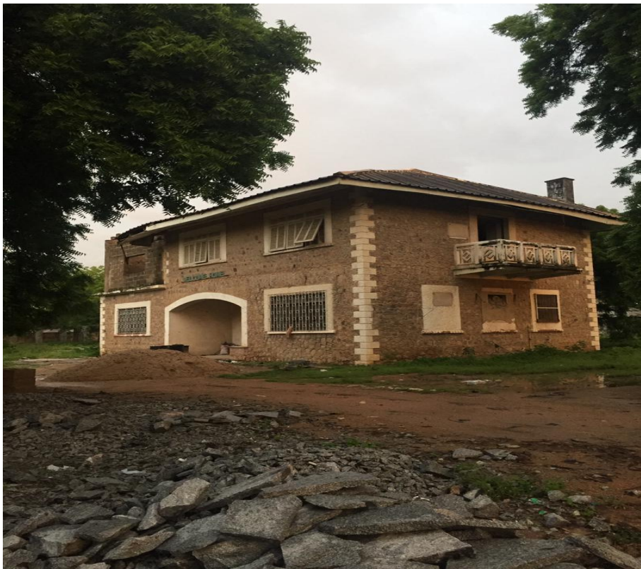
Figure 5: A British Colonial Building located at Lodge Road, Nassarawa GRA
